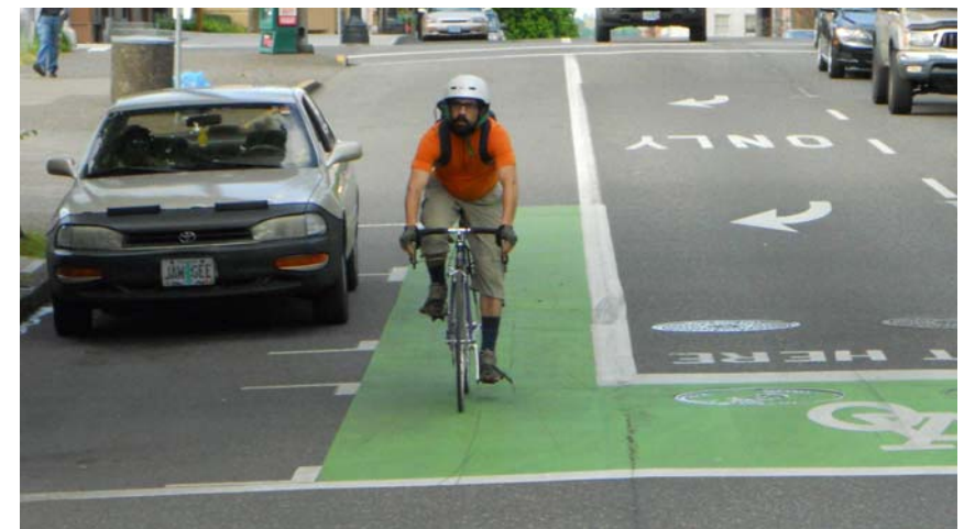
COLORLED BIKE BOX RESTRICTS RIGHT TURNS ON RED AND PROVIDES A SAFE REFUGE FOR CYCLISTS. RECOMMENDED BIKE BOX LOCATIONS ARE SYMBOLIZED AS B ON PAGE 110
