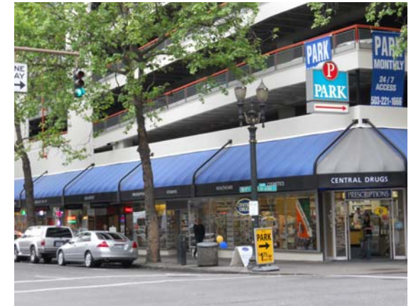
GROUND FLOOR RETAIL IN THIS PARKING STRUCTURE ACTIVATES THE STREET; AWNINGS PROVIDE WEATHER COVER
