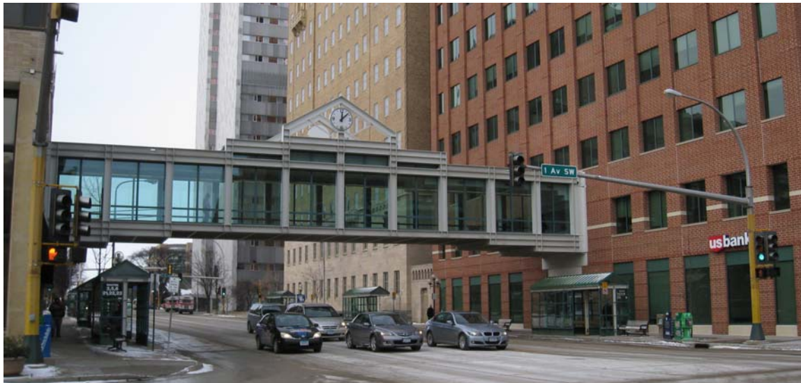
SKYBRIDGE OVER 2ND STREET
