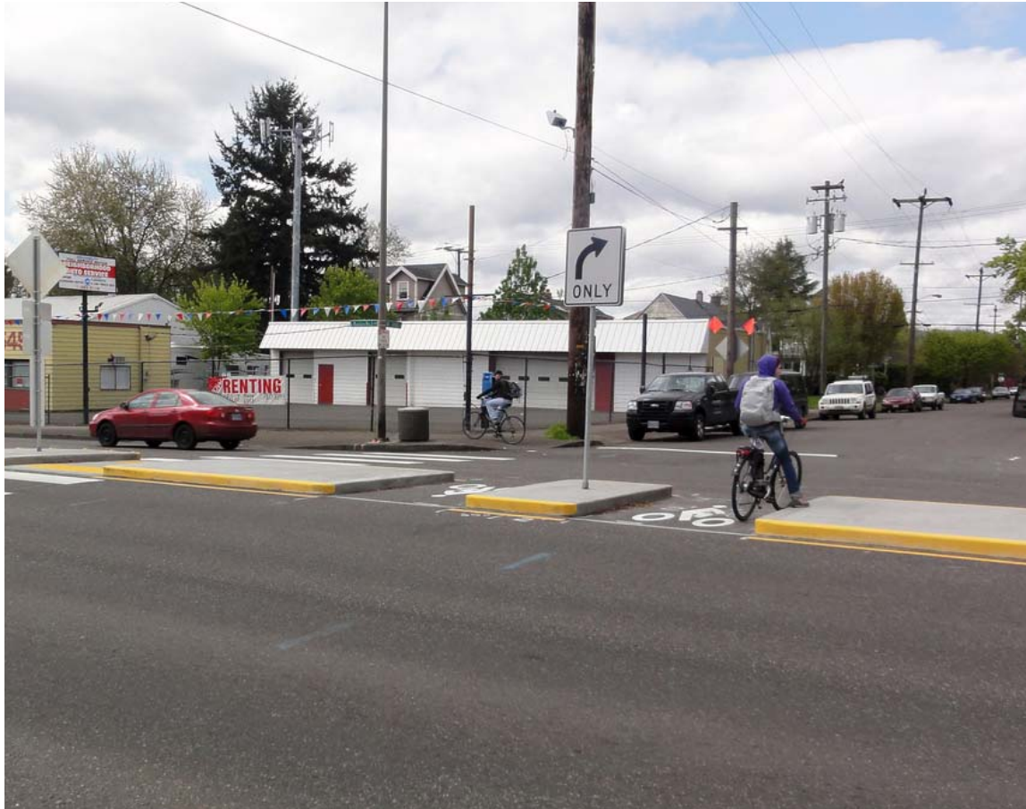
REFUGE MEDIANS ALLOW FOR SAFER CROSSINGS AT LARGER, HIGH SPEED INTERSECTIONS. RECOMMENDED LOCATIONS FOR BICYCLE AND PEDESTRIAN REFUGE MEDIANS ARE SYMBOLIZED AS D AND E ON THE MAP ON PAGE 110
