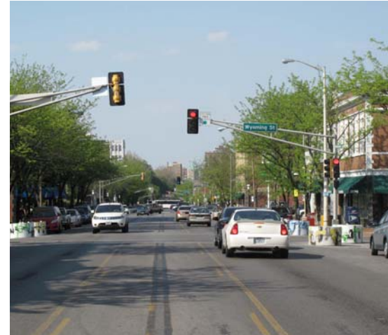
TRAFFIC CALMING PROJECT IN ST. LOUIS USING A LANE REDUCTION PLANTERS THAT ACT AS CURB EXTENSIONS
