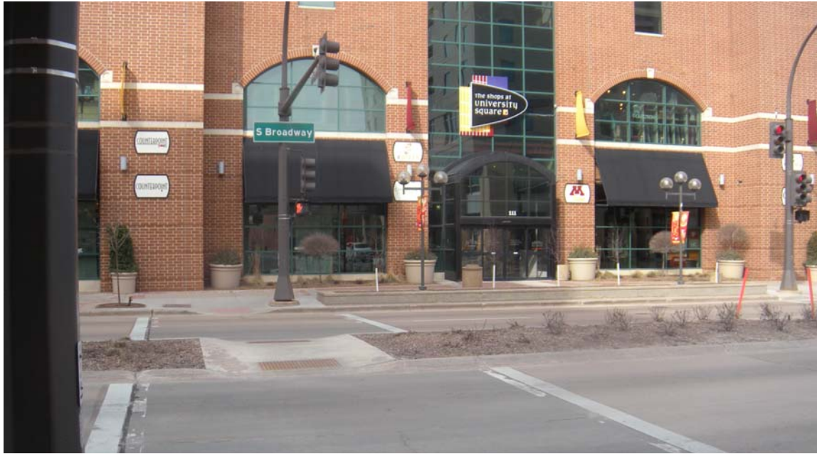
THE CROSSING OF BROADWAY AT 1ST STREET S OFFERS A PEDESTRIAN ACTIVATED SIGNAL AND A MEDIAN REFUGE TO REDUCE CROSSING DISTANCE AND EXPOSURE
