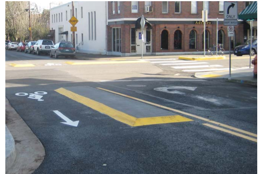
BICYCLE BOULEVARD TREATMENTS ALLOW THROUGH BIKE MOVEMENTS WHILE RESTRICTING VEHICLES FROM TRAVELING THROUGH THE INTERSECTION. A SIMILAR TREATMENT IS RECOMMENDED AT LOCATION A ON THE MAP ON PAGE 110
