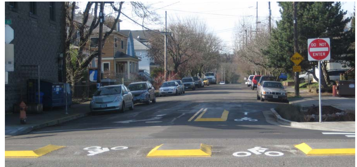
MEDIAN ALLOWING THROUGH BICYCLE TRAFFIC RECOMMENDED FOR 3RD AVENUE AT 6TH STREET SOUTH
