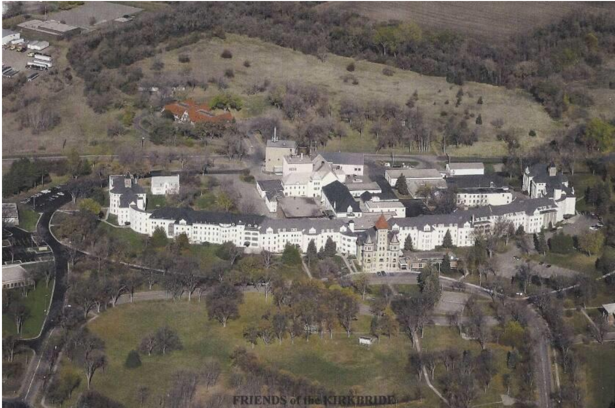
Aerial image of the Kirkbride Plan Fergus Falls State Hospital. Image via The Forum (Fargo-Moorhead), https://www.inforum.com/newsmd/fergus-falls-landmarks-future-in-doubt .
