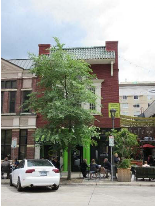
Rochester Commercial Club Building, west façade, facing east, 2017, PVN.
