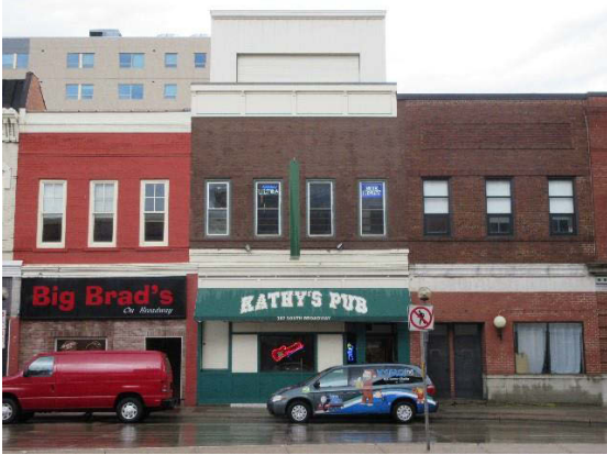
Clausen and Adler Hardware, east façade, facing west, 2017, PVN.
