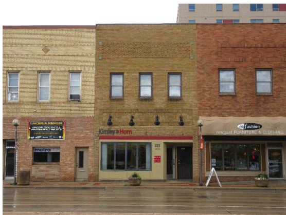
Commercial Building, east façade, facing west, 2017, PVN.
