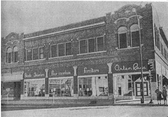
Riverside Building, north façade, c. 1946 – 1957, image courtesy of the Rochester Heritage Preservation Commission.
