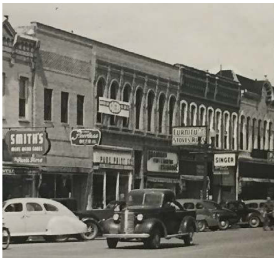
Black's Lunch east façade, facing northwest, 1940, image courtesy of the Rochester Heritage Preservation Commission.
