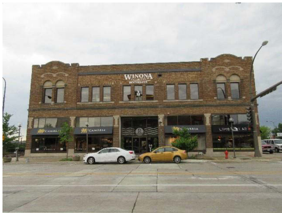
Riverside Building, north façade, facing south, 2017, PVN.
