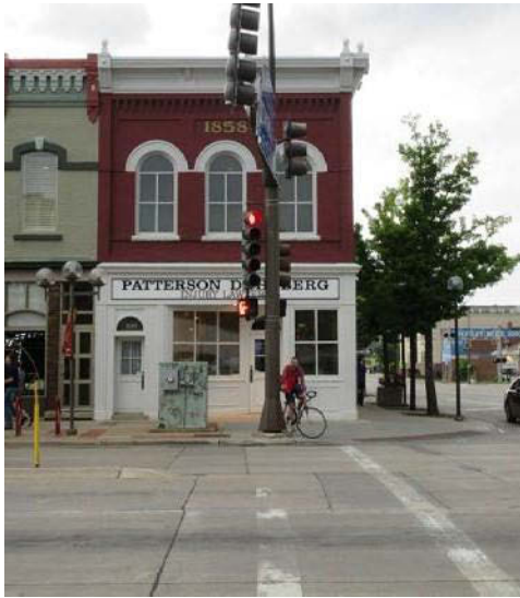
Commercial Building, west façade, facing east, 2017, PVN.
