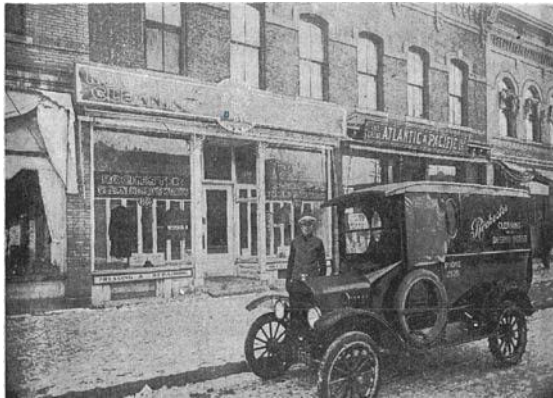
Great Atlantic & Pacific Tea Co. west façade, facing southeast, c. 1920, image courtesy of the Rochester Heritage Preservation Commission.
