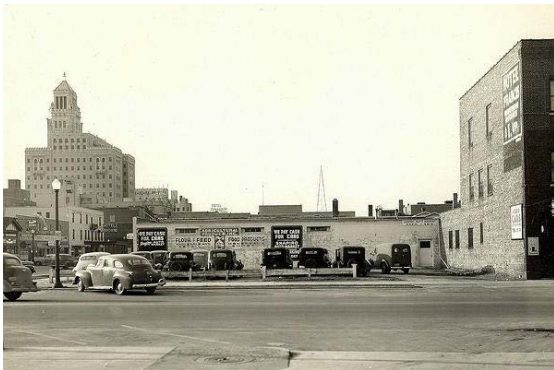
Commercial Building, south façade, facing north, c. 1940s, image in Lee Hilgendorf and Cindy Scott, "Photos: Lens on History," June 29, 2017, (Rochester) Post-Bulletin.
