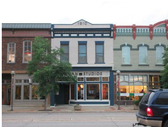
C.H. Morrill and Son Wholesale Grocer, west façade, facing east, 2017, PVN.
