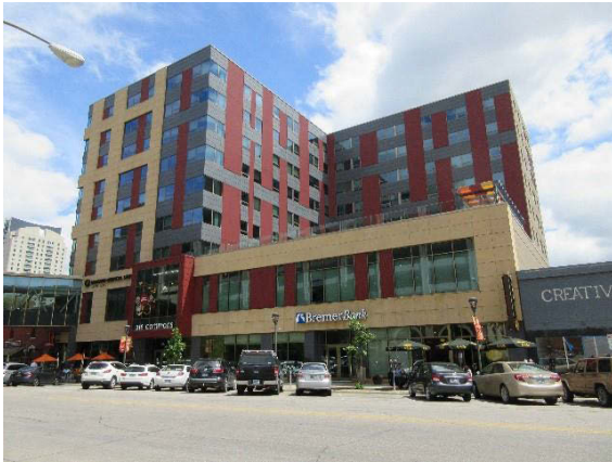
318 1 st Avenue South, west façade, facing northeast, 2017, PVN.
