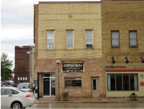
F.A. Poole Building, east façade, facing west, 2017, PVN.
