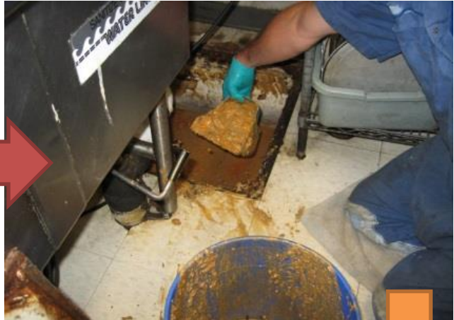
Remove grease from top
