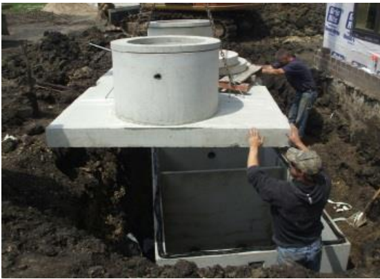
Figure 2: Gravity grease interceptor
