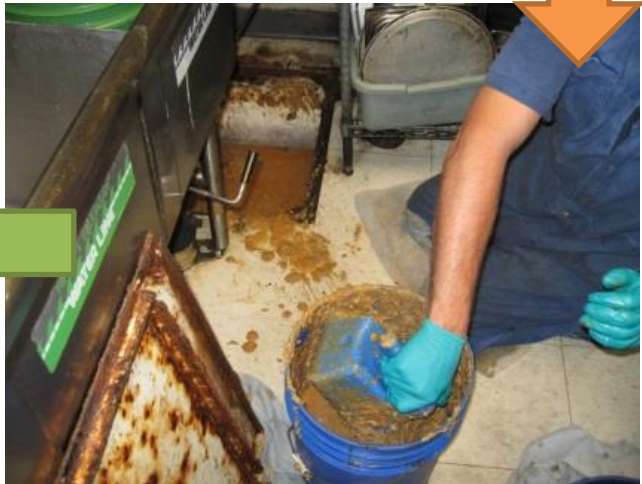
Remove solids from bottom
