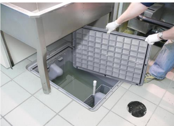
Figure 3: Hydromechanical grease interceptor
