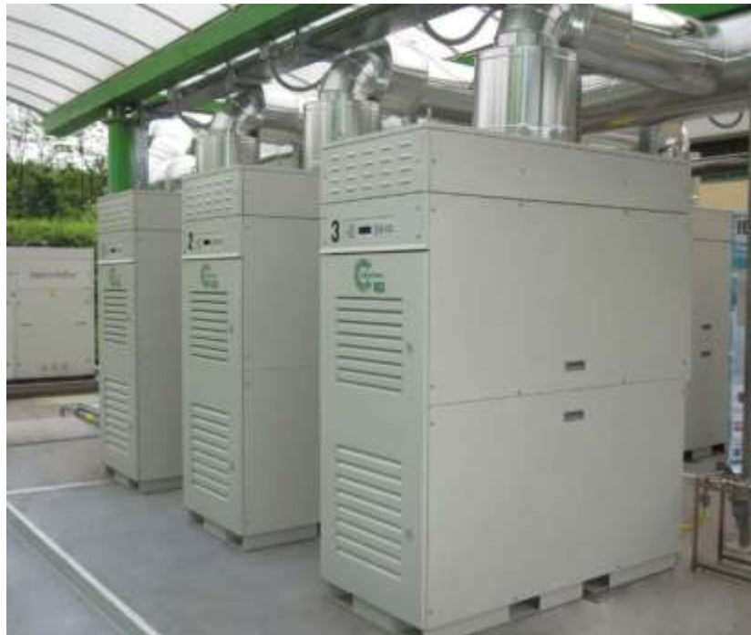
Figure 2-3. Example microturbine installation with integrated exhaust manifold
