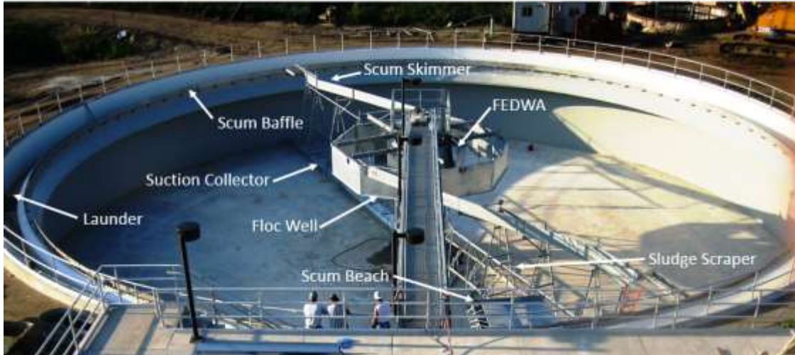
Figure 2-2. Final Clarifier 5 arrangement
