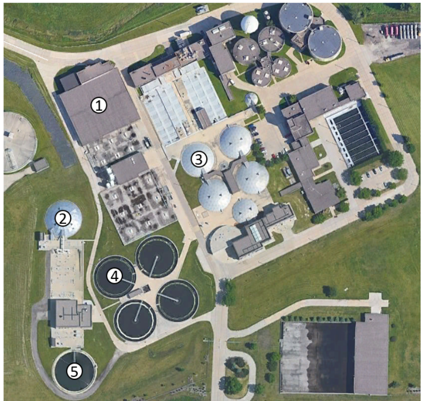
Figure 1-1. Rochester WRP Aerial View
