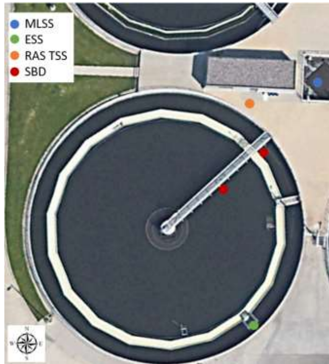
Figure 3-5. Final Clarifier 3 stress test sample locations
