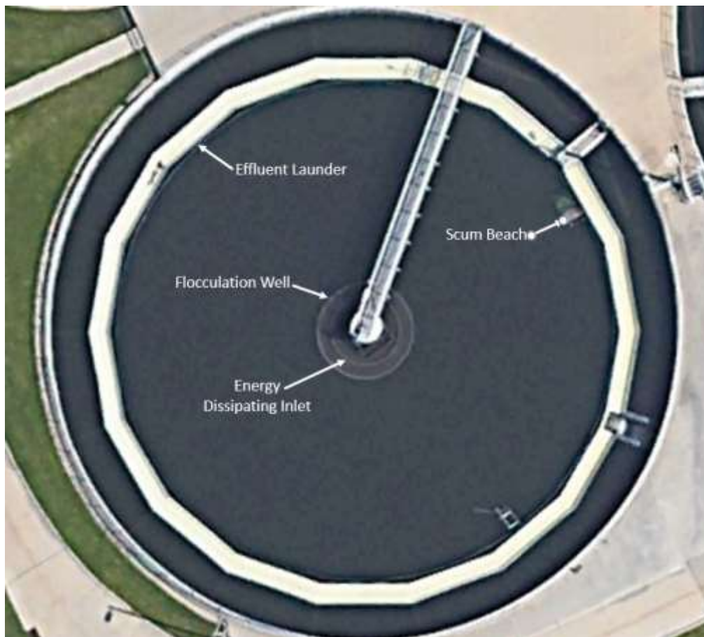
Figure 3-3. Final Clarifiers 1-4 configuration
