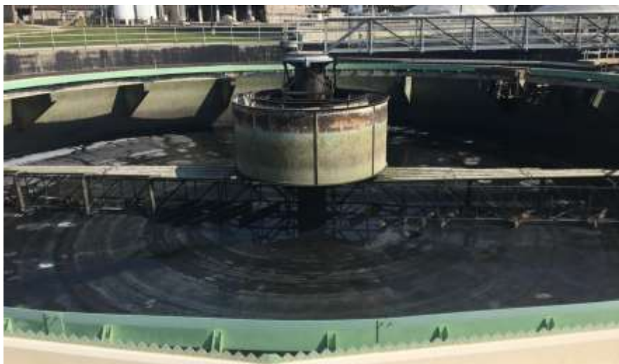
Figure 3-4. Final Clarifier 1-4 organ pipe sludge collector
