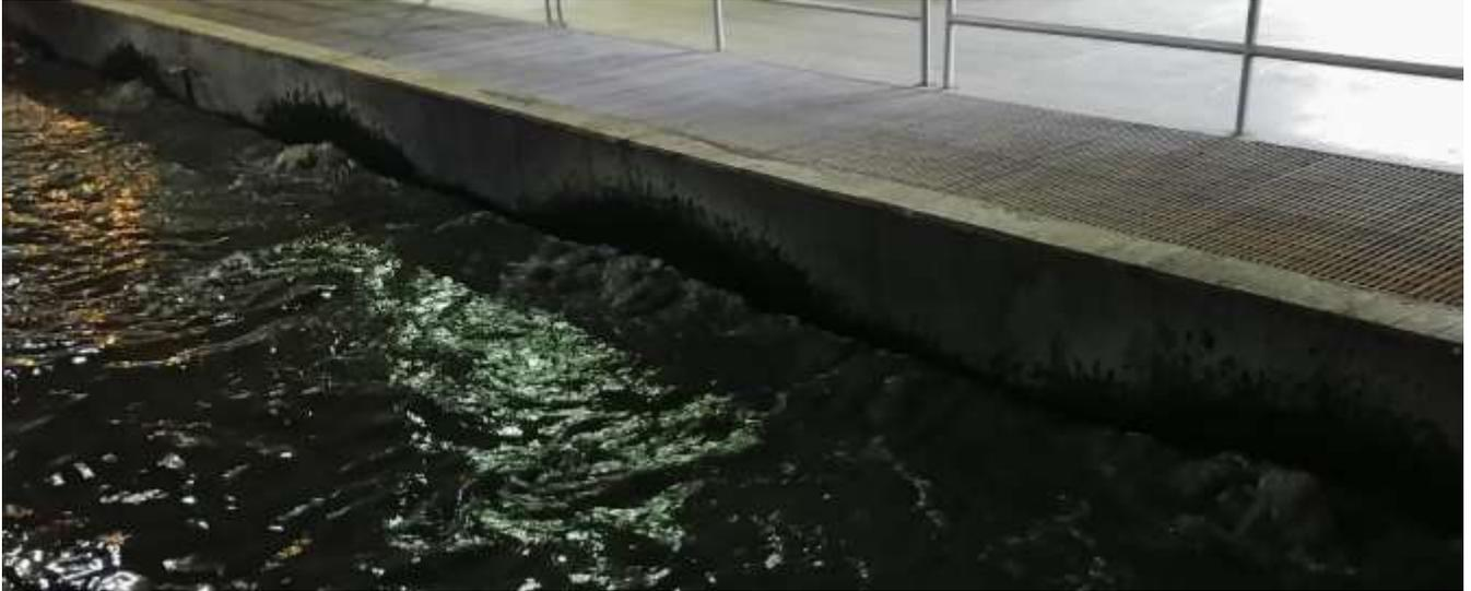
**Figure 2-12. Inlets during high flows of stress test**
