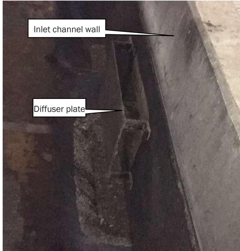
Figure 4-9. Existing diffuser plate photograph
