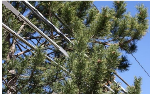
Figure 4. Branches touching power line From: photos-public-domain.com
