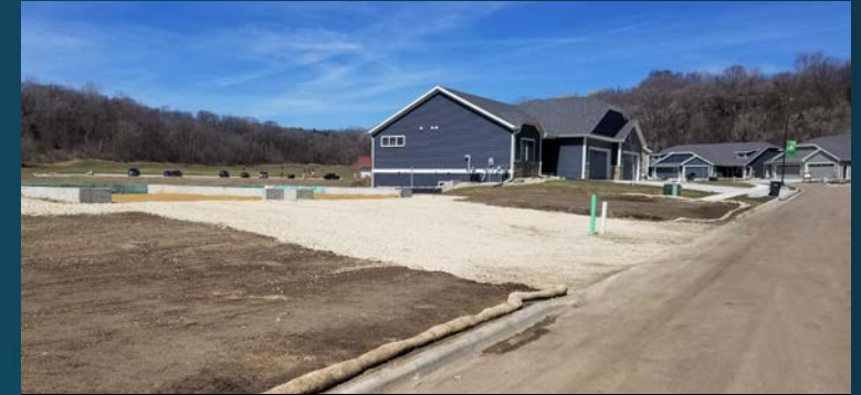
Residential Subdivision ESC Inspection
