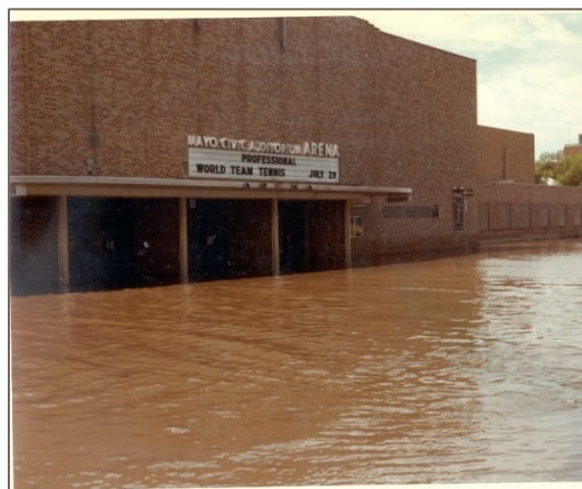
Impact of the 1978 Flood on the Mayo Civic Center
