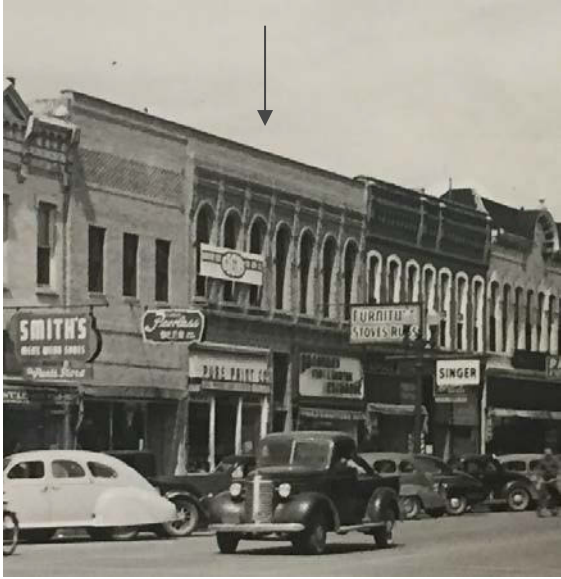
The Baker and Hanson/Council Saloon Building, east façade, facing northwest, 1940, image courtesy of the Rochester Heritage Preservation Commission.
