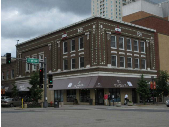
I.O.O.F. Lodge #13, west and south façades, facing northeast, 2017, PVN.
