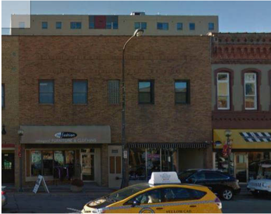
The Baker and Hanson/Council Saloon Building, east façade, facing west, 2017, PVN.
