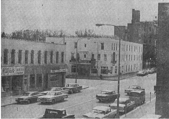
Williams block, north façade, facing southwest, c. 1960s, image courtesy of the Rochester Heritage Preservation Commission.
