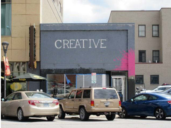
Commercial Building, west façade, facing east, 2017, PVN.
