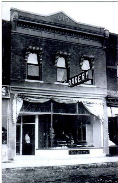
C.H. Morrill and Son, Wholesale Grocer,, west façade, facing southeast, c. 1910, image in Rochester by Alan Calavano.
