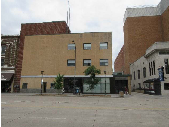
Northwestern National Bank of Rochester, south façade, facing north, 2017, PVN.
