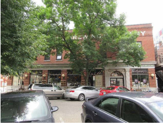
Union National Bank Building, north façade, facing south, 2017, PVN.
