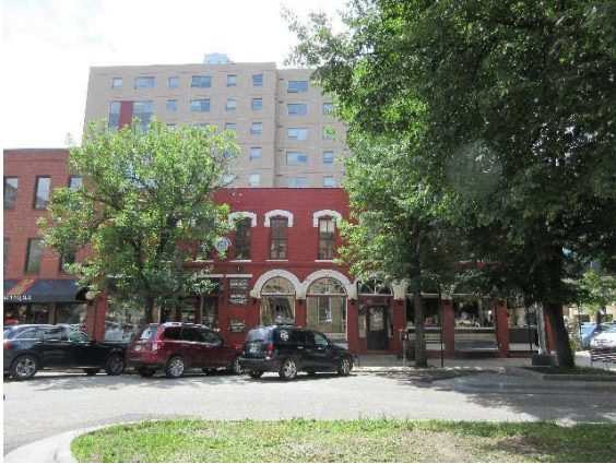
Williams Block, north façade, facing south, 2017, PVN.
