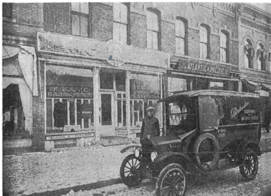
Great Atlantic & Pacific Tea Co. west façade, facing southeast, c. 1920, image courtesy of the Rochester Heritage Preservation Commission.
