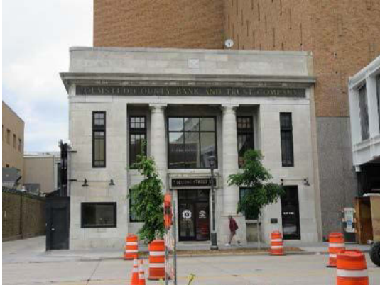
Olmsted County Bank and Trust Company, south façade, facing north, 2017, PVN.
