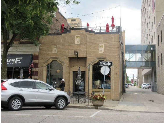
Lawler Laundry Building Façade, north façade, facing south, 2017, PVN.
