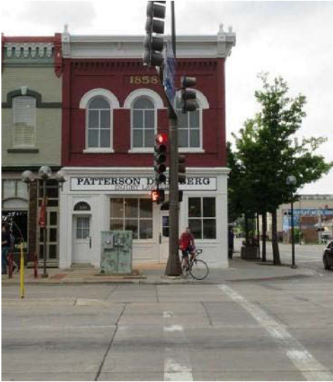
Commercial Building, west façade, facing east, 2017, PVN.
