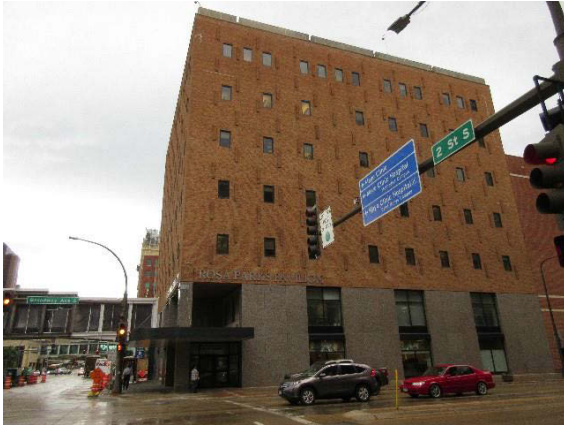
Dayton's Department Store, east façade, facing west, 2017, PVN.
