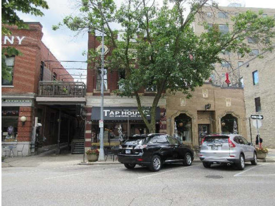
Kennedy Building, north façade, facing south, 2017, PVN.
