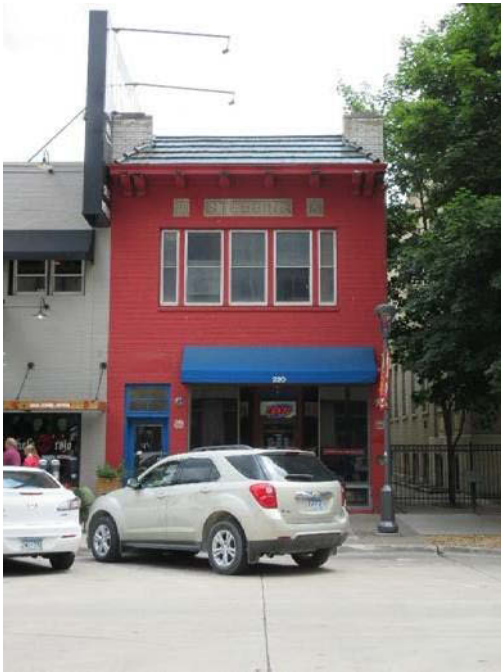
Stebbins Building, west façade, facing east, 2017, PVN.
