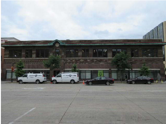
C. F. Massey Co., north façade, facing south, 2017, PVN.
