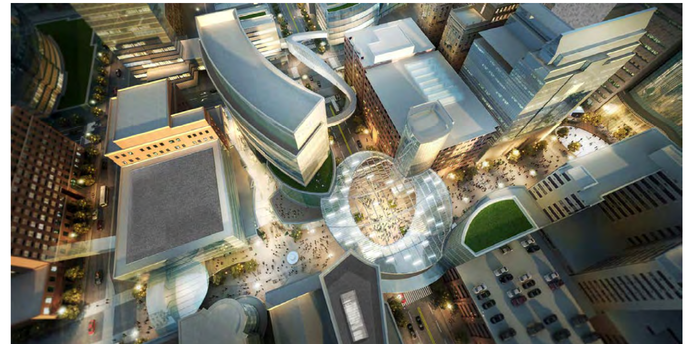
A vision for significant commercial development, signature streets, and public spaces in the Heart of the City area of downtown Rochester.
