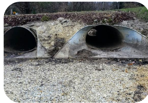
Outfall Pipe Cleanings
