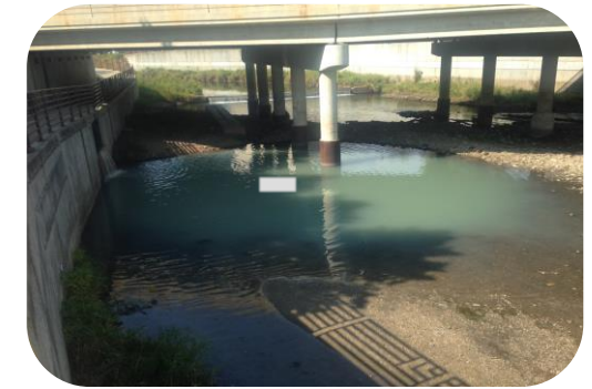
Process water from Seneca facility
