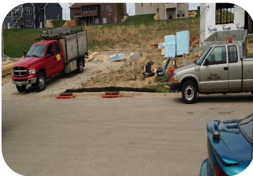
Inlet Protection Compliance
