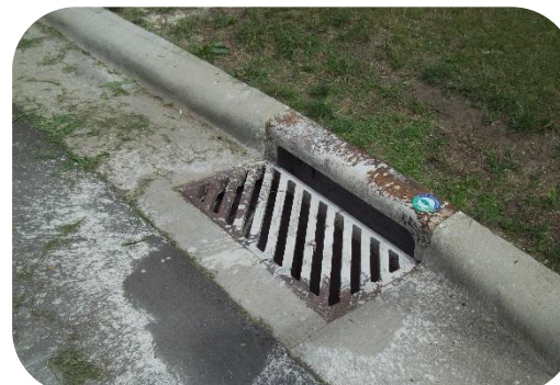
Concrete washout to catch basin
