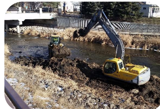
Sediment Removal from Zumbro River
