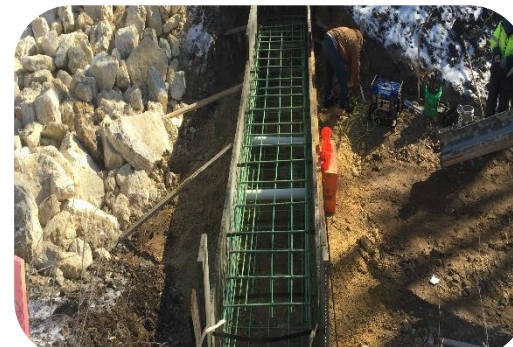
Rocky Creek Channel Restoration Project
