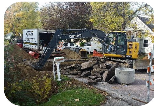
Storm Sewer Replacement
