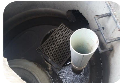
SAFL Baffle HydroDynamic Separator
