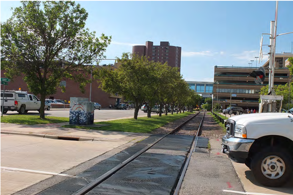
View of CP Rail spur line looking south.
