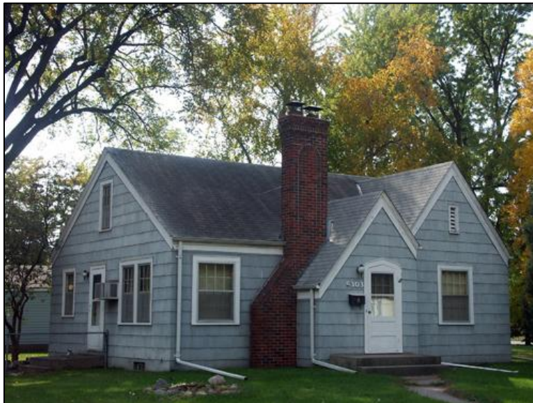
Figure 11. Minimal Traditional. Minneapolis, Minnesota
