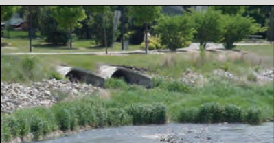
Storm Water Management
