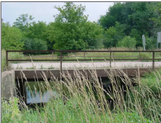
Downstream of bridge
