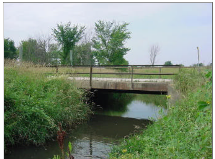
Upstream of bridge
