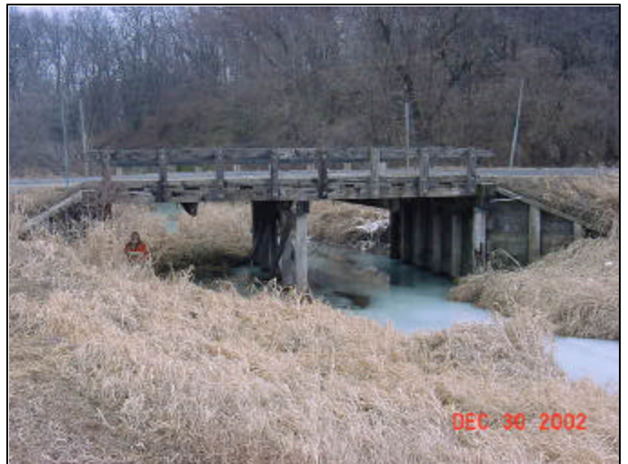
Upstream from bridge
