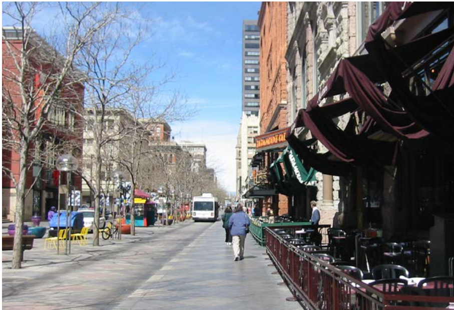
Representative Shared Street. The curbless design and cohesive paving materials allow for flexible usage ultimately catering to pedestrians and bicyclists.
