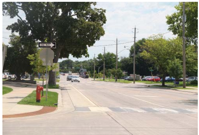
Existing Conditions: 6th St. SW & 3rd Ave SW
