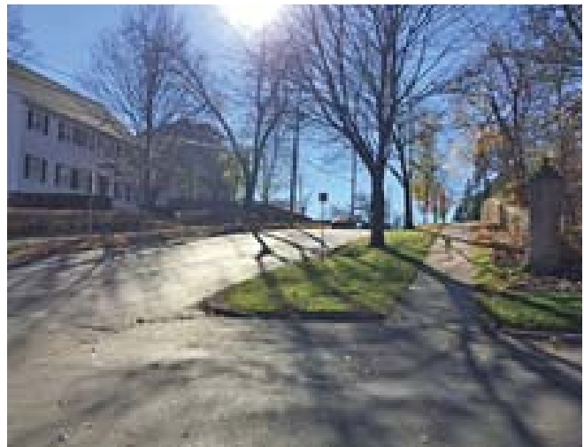
View of steep gradient and retaining walls on 7th Ave SW
