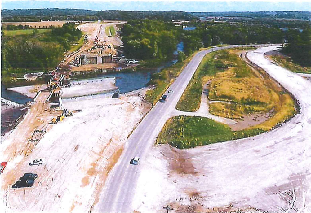
Construction of the new 55th Street Northwest bridge in Rochester.
