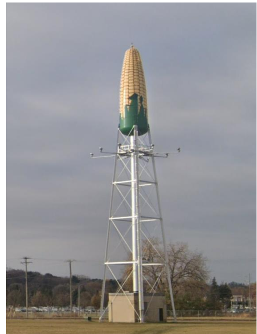
Ear of Corn Water Tower - from 3 rd Avenue. (Image is looking west/southwest) xviii
