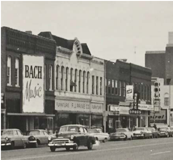
F.J. Paine Co./Palace Block, east façade, facing northwest, c. 1965, image courtesy of the History Center of Olmsted County, detail of "Street Scene" 2005.105.040.
