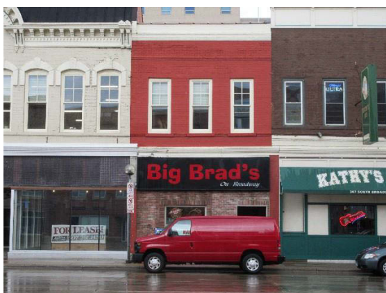
F.J. Paine Co., east façade, facing west, 2017, PVN.
