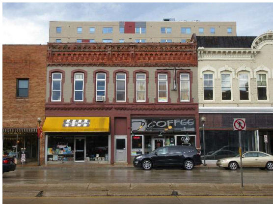
Bach Music Company, east façade, facing west, 2017, PVN.
