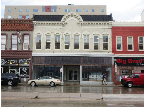
F.J. Paine Co./Palace Block, east façade, facing west, 2017, PVN.
