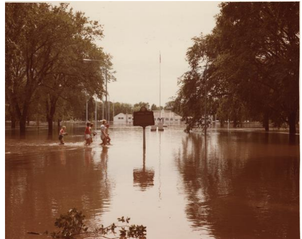
“View of Flooding”, July 6, 1978 20
