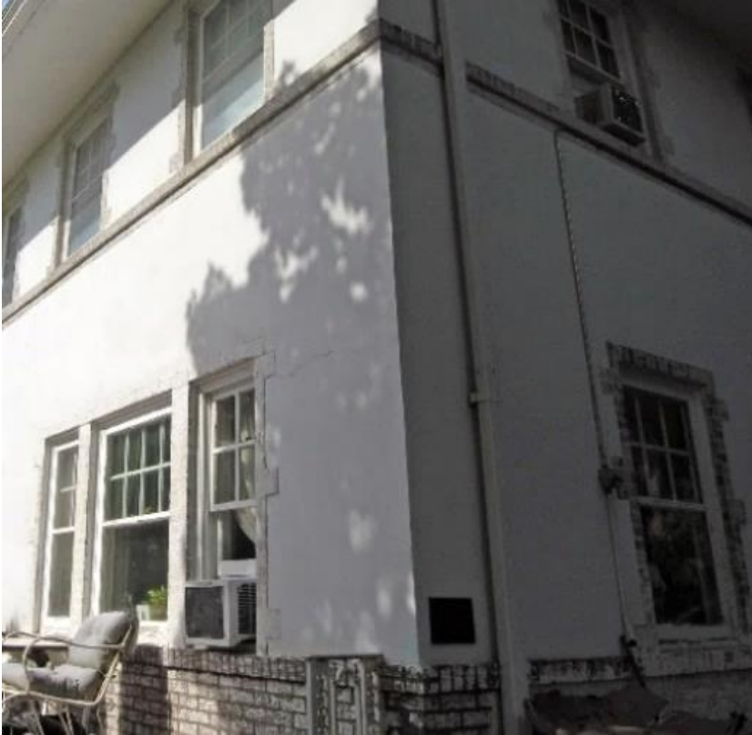
Brick-clad foundation & bands at northeast corner, looking southwest
