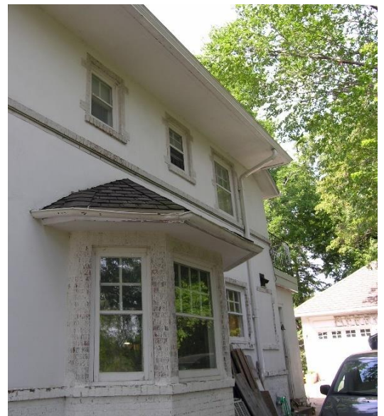
North elevation (detail), looking southwest
