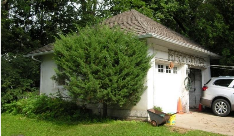
Garage, south and east elevations, looking northwest
