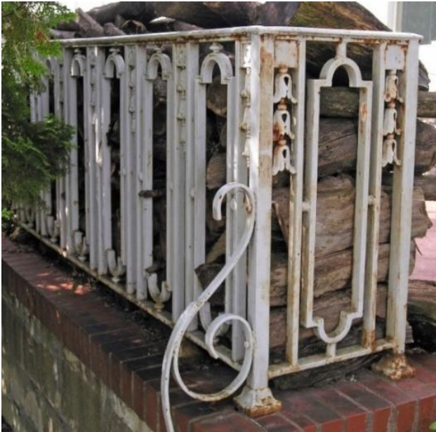
Iron terrace balustrade at east façade
