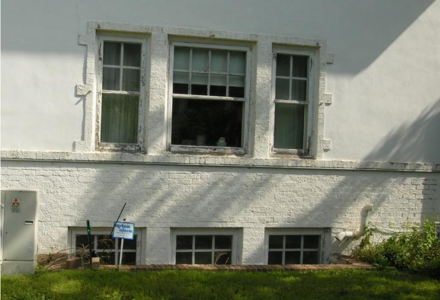
Horizontal groupings of windows at south façade, looking north
