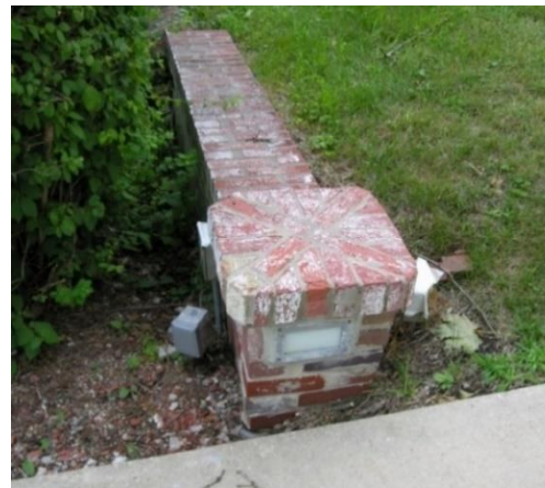
Retaining wall at driveway, looking south 1
