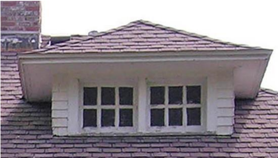
Window with horizontal orientation at west elevation, looking east
