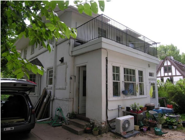
Single-story projection at west façade, looking southeast
