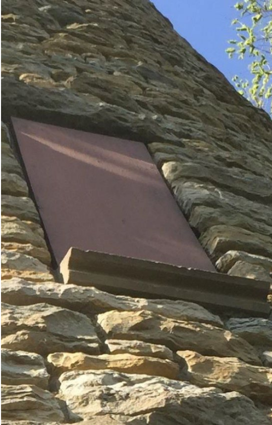
Existing condition of boarded tower windows, typical.
