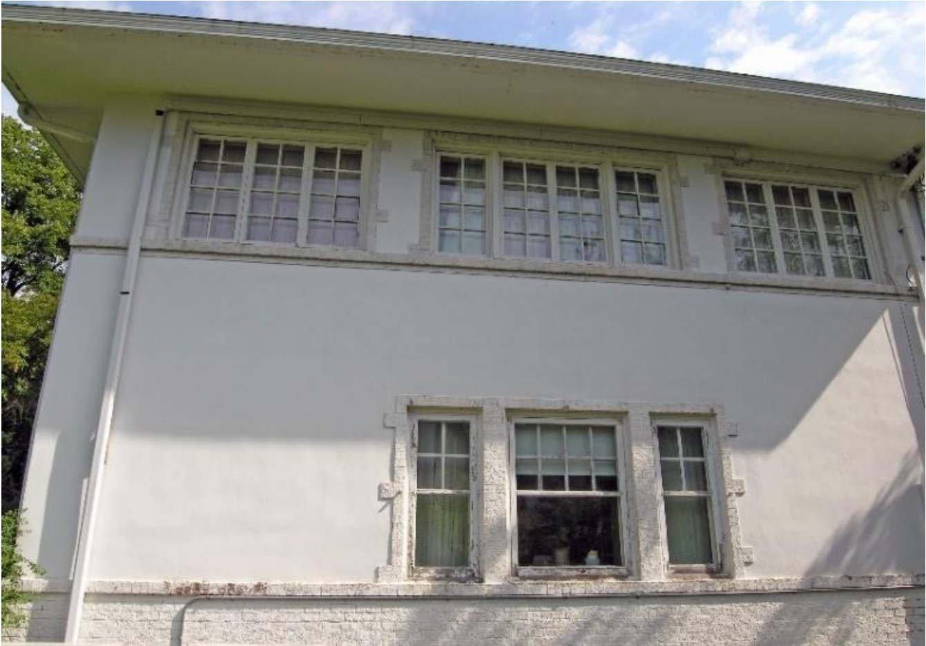
South elevation, looking north
