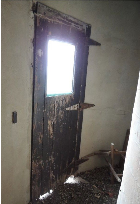
Existing condition of the doors, typical.
