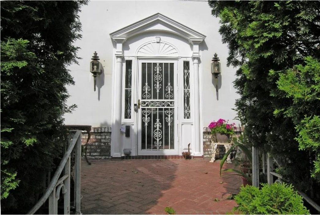
Front door detail, looking west
