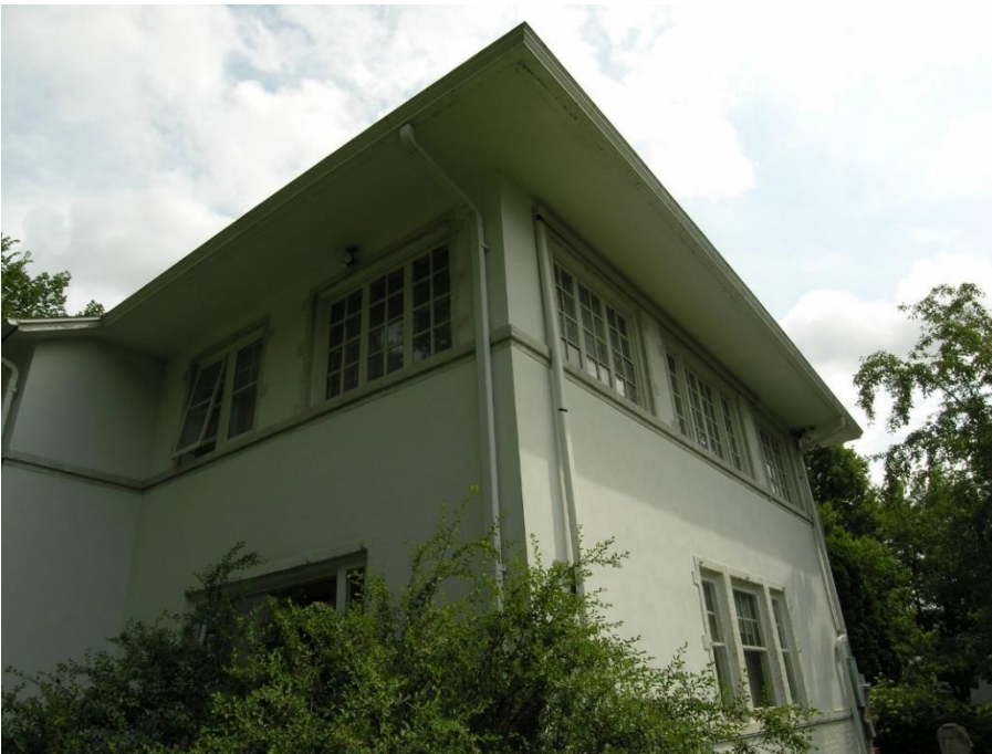
Ribbon of windows, second floor of west & south façades, looking northeast
