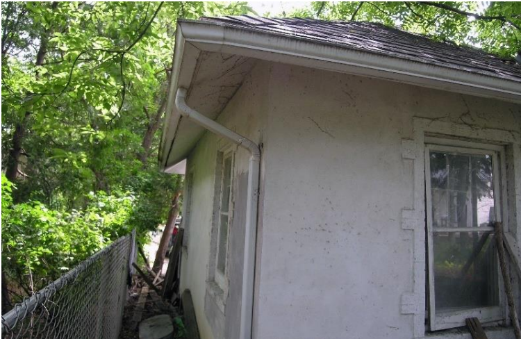
Garage, north and west elevations, looking southeast
