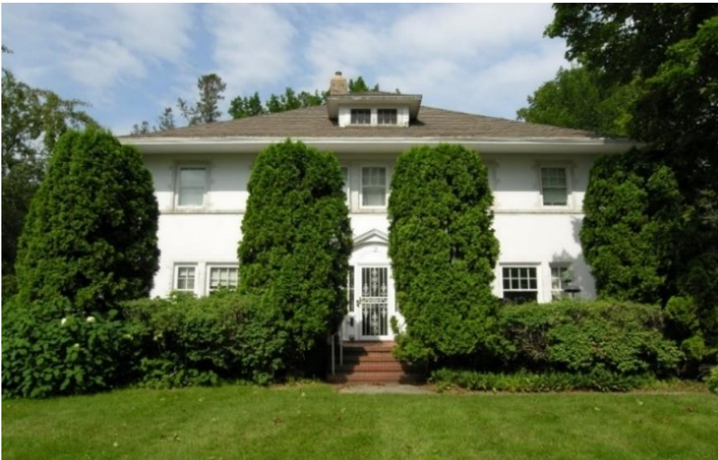
East elevation, looking west
