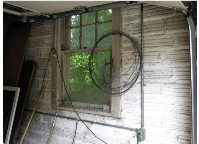
Garage interior, structural clay tile, looking northwest
