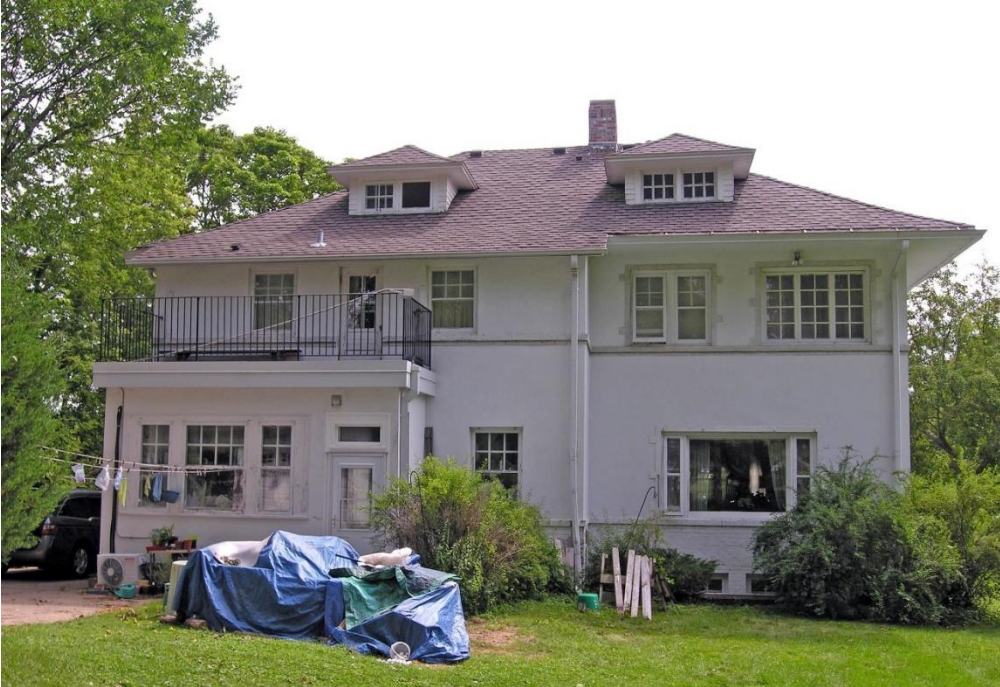
Roof and dormers at west façade, looking east
