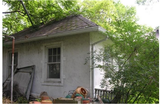
Garage, west and south elevations, looking southeast
