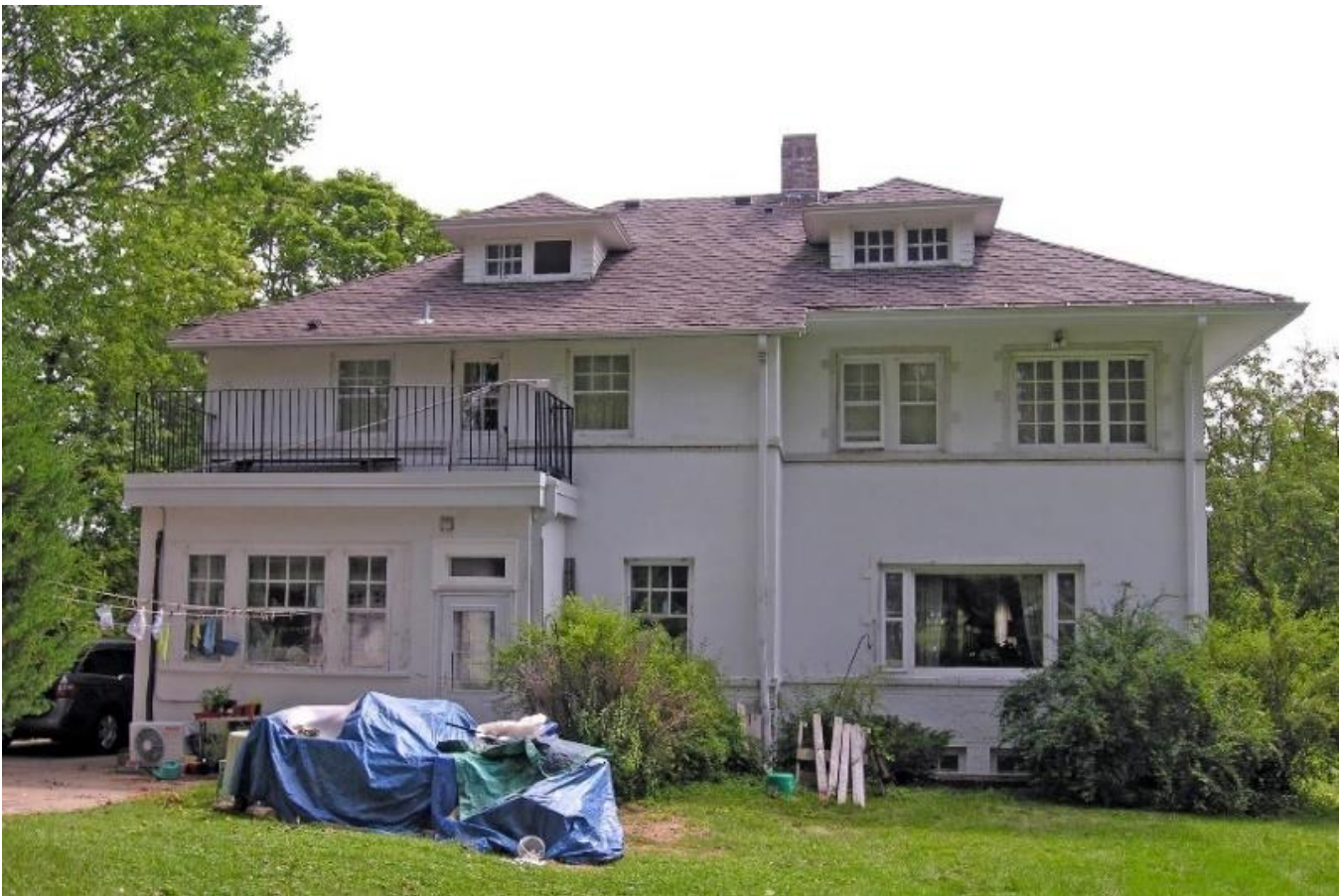
West elevation, looking east
