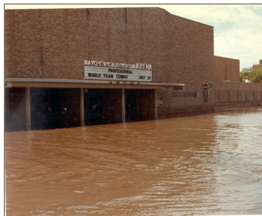
Impact of the 1978 Flood on the Mayo Civic Center
