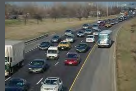
At-Grade, Dynamic Shoulder
